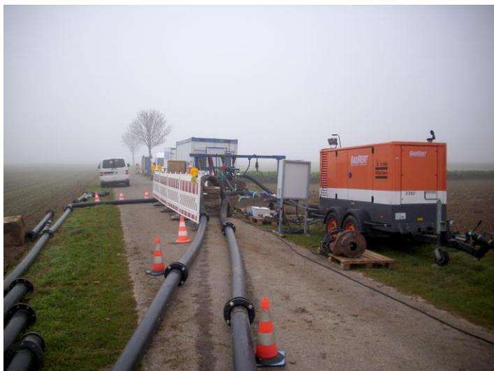
During the work on sewers in Bad Fallingbostel, the waste water had to be partly conveyed above ground more than 3,000 metres to the nearest junction. Due to the fluctuating dry matter content, a TORNADO® rotary lobe pump from NETZSCH was used.
